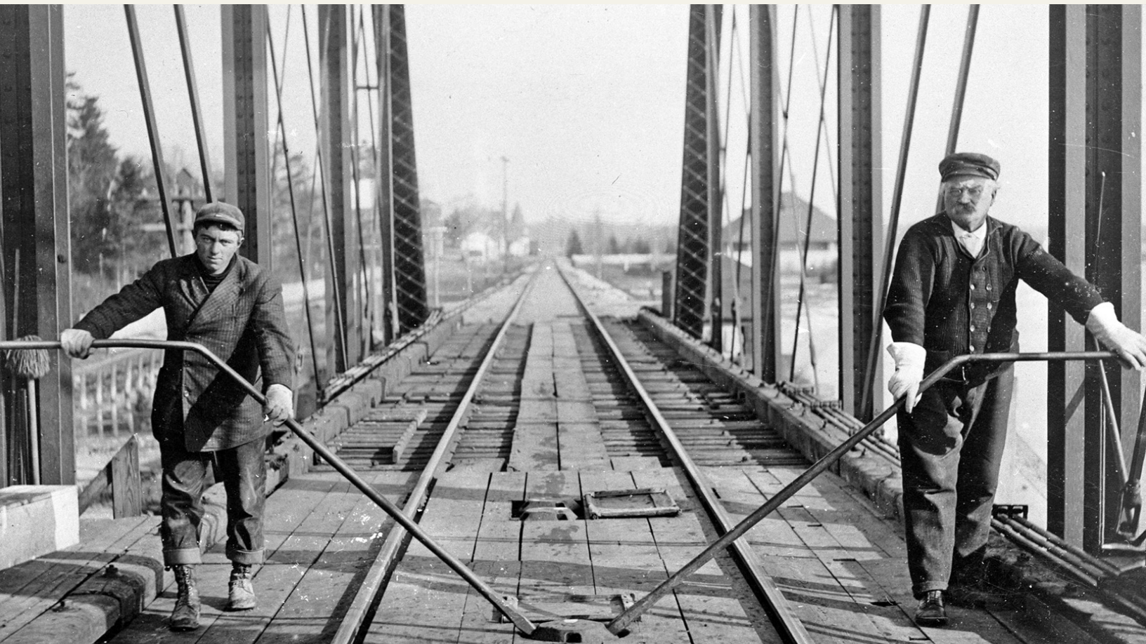
Charlevoix bridge tenders manually turning the railroad bridge with 'keys,' later replaced by electricity.
