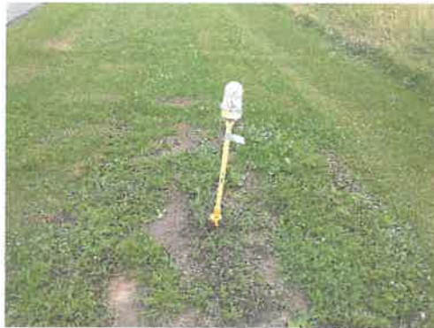
Typical Edge Light Installation at Sanderson Field
