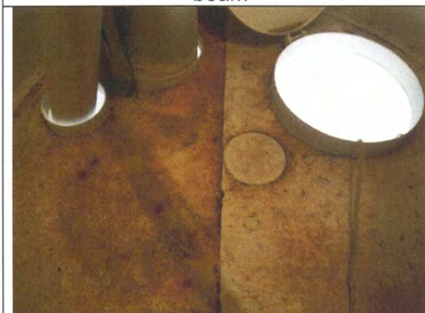
Corrosion on condensate platform
