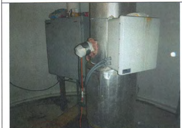
Fill pipe, expansion joint and controls
