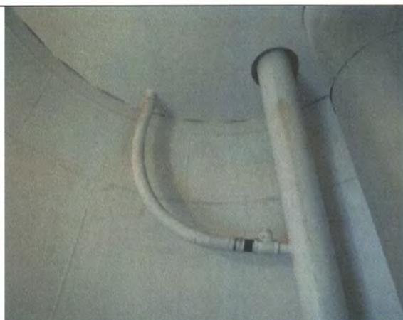
Condensate drain hose connection to overflow pipe
