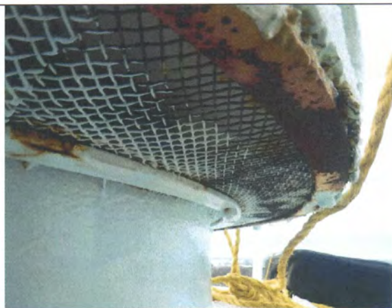
Access tube vent screen and bands
