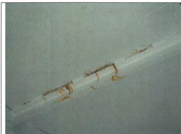
Corrosion at condensate platform support beam
