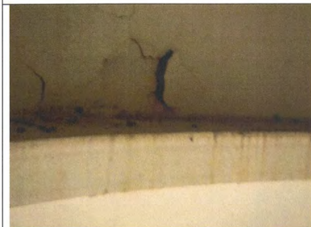
Lifting at pedestal stiffener ring
