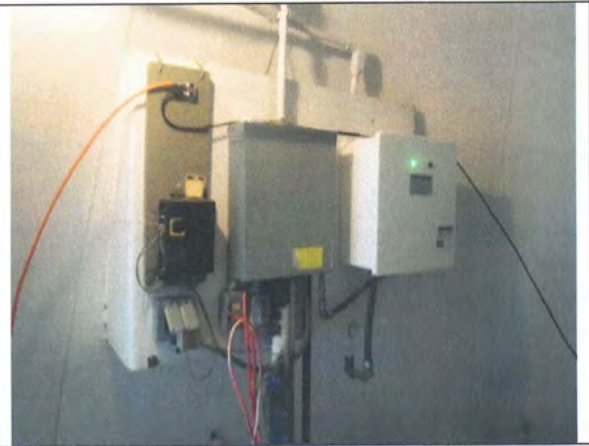
Cathodic protection and electric panels
