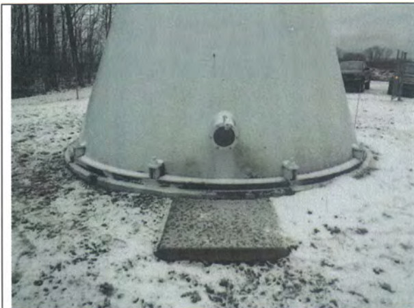
Overflow pipe and splash pad
