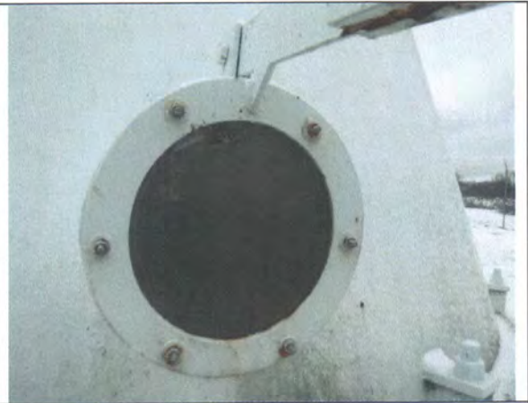
Overflow pipe flap gate with 24-mesh screen
