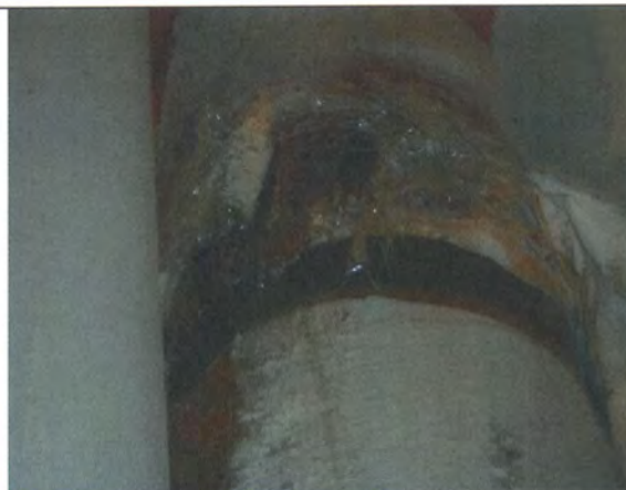
Damage to fill pipe insulation at upper pedestal
