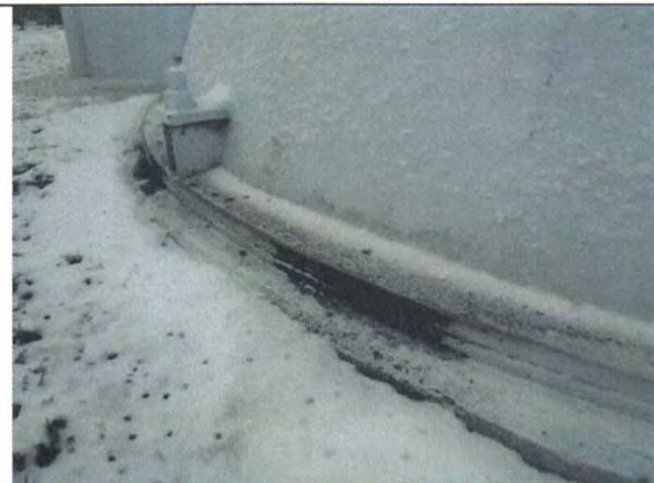
Typical view of foundation and grout
