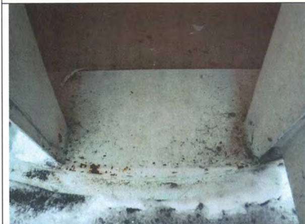
Minor coating breaks at basebell entrance
