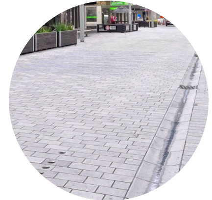
SPECIALTY PAVEMENT (POTENTIAL): textured or pervious pavement reinforces the pedestrian-priority nature of the street, potential environmental benefits, flush curb maximizes accessibility, tactile strips at entrances to shared roadway
