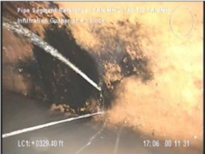
MH 2-147 to MH 2-146 Infiltration, cracks
