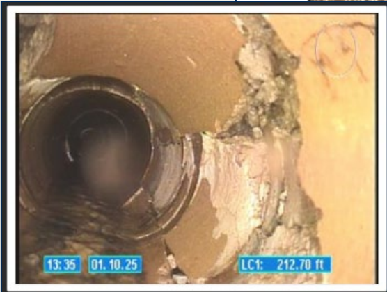
MH 2-118 to MH 2-120 Infiltration at joints
