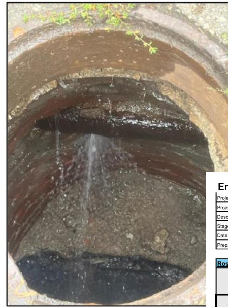
Figure 1. Water main in a sanitary manhole on Bond Street.
