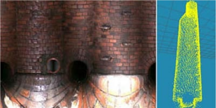
MH 2-118 to MH 2-120 Infiltration at joints
