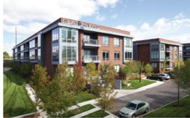
Image: Multi-Unit Building
