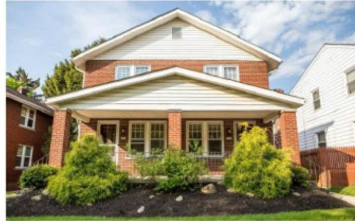
Image: Duplex Building
